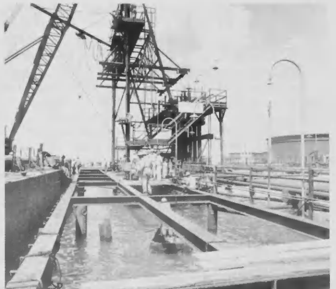
Small boats, as seen in the foreground, and frogmen handle the work under the steel structures of West Pier. Botonan chikito, manera esun aki dilanti, y buzadornan ta traha ariba e estructuranan di stal di West Pier.
